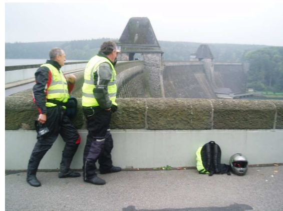
Where did we make the hole...??
